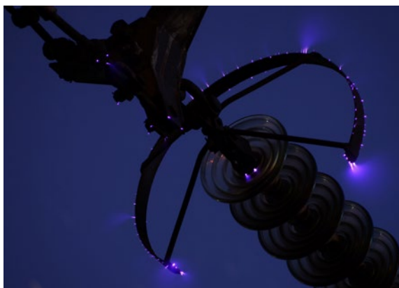
Figure 2: A corona discharge on an insulator string of a 500 kV overhead power line. Image by Nitromethane , own work, CC BY-SA 3.0
